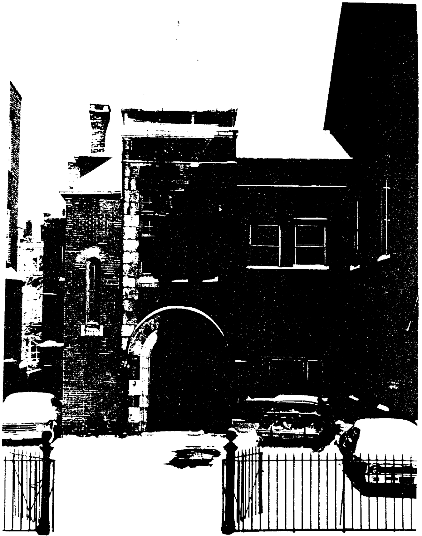
SOUTH CONGREGATIONAL CHURCH LADIES PARLOR AND SUNDAY SCHOOL 267 President Street Built 1889
