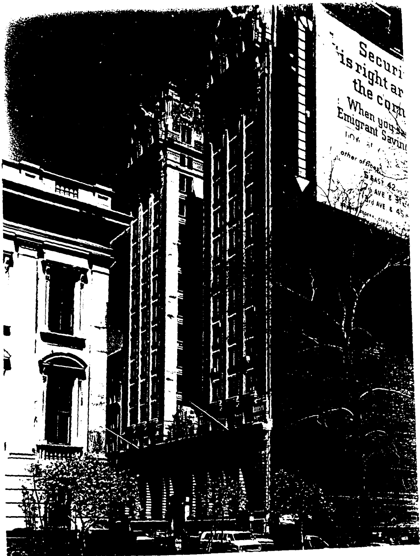
Former Emigrant Industrial Savings Bank Building 51 Chambers Street, Manhattan
