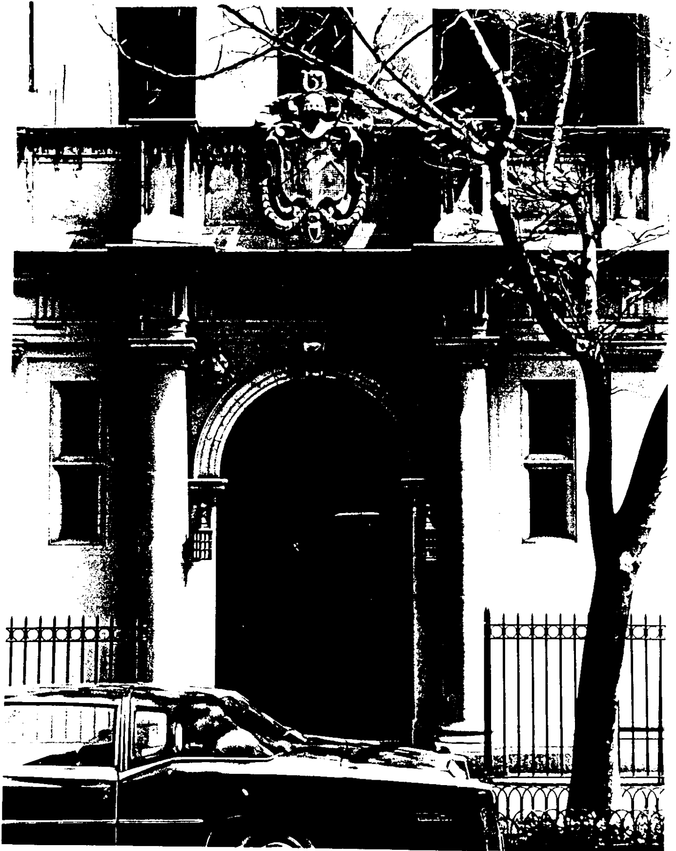
1025 PARK AVENUE HOUSE Front entrance detail
