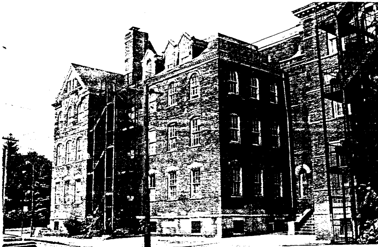
P.S. 20 Annex Heberton Avenue elevation (east) of the 1891 building Photo: Carl Forster
