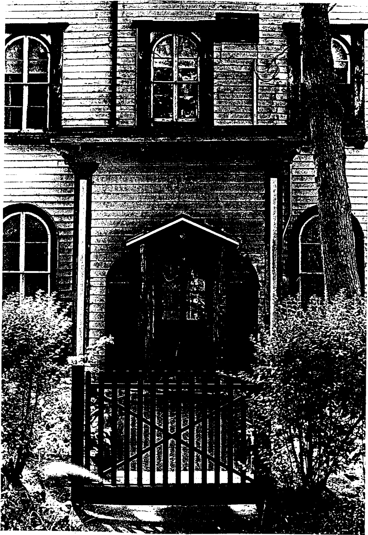
GUSTAVE MAYER HOUSE - Rear (Northwest) Elevation, Detail
