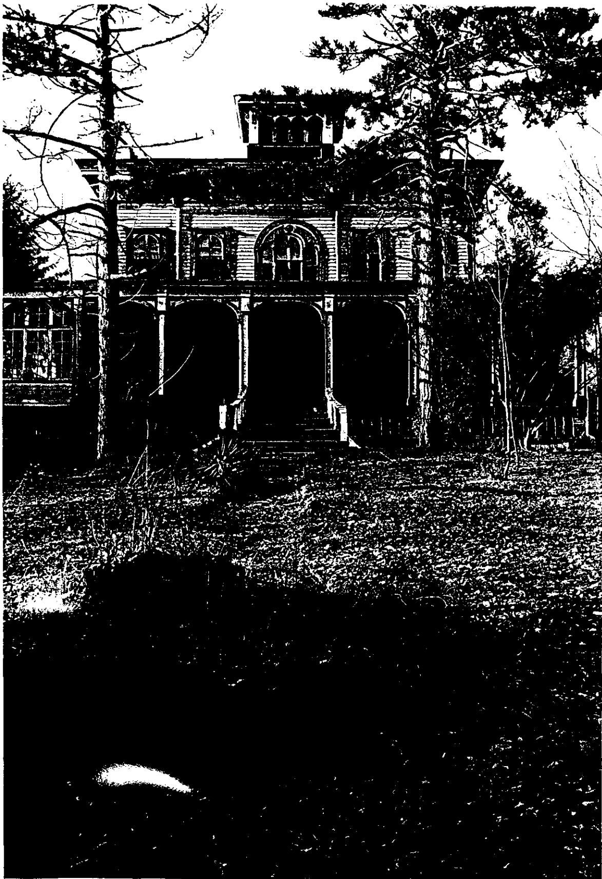
GUSTAVE MAYER HOUSE - Front (Southeast) Facade
