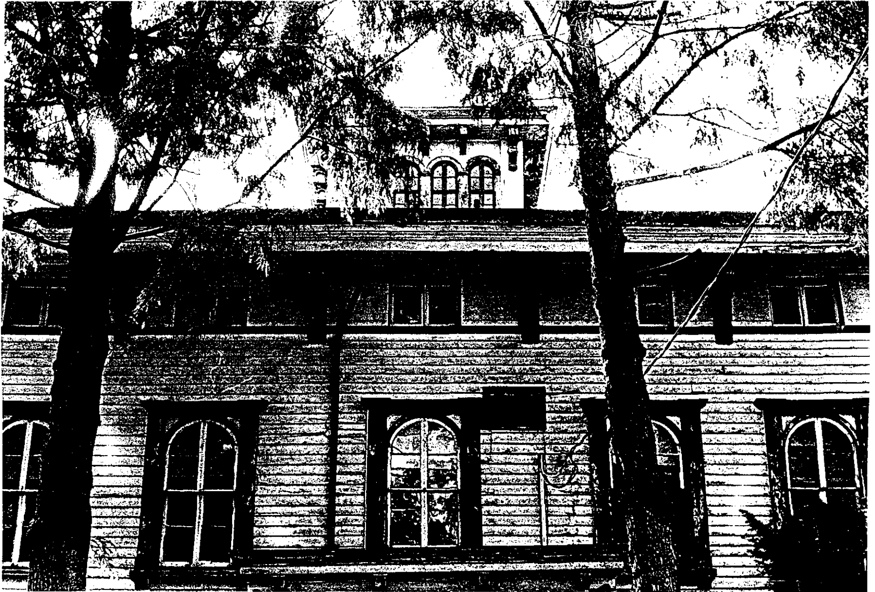
GUSTAVE MAYER HOUSE - Rear (Northwest) Elevation, Detail
