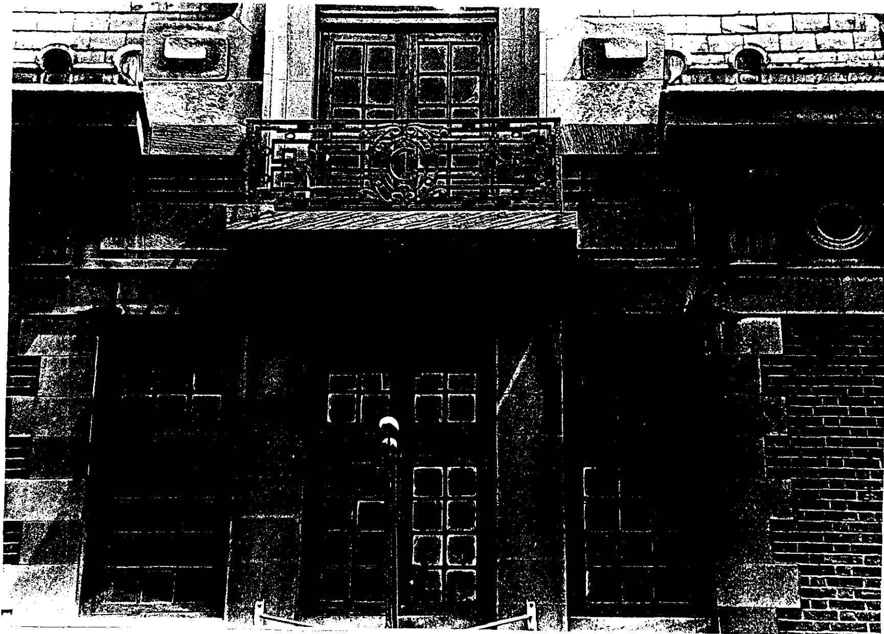
Plate 3. Detail, third and fourth stories, 213 West 58th Street.
