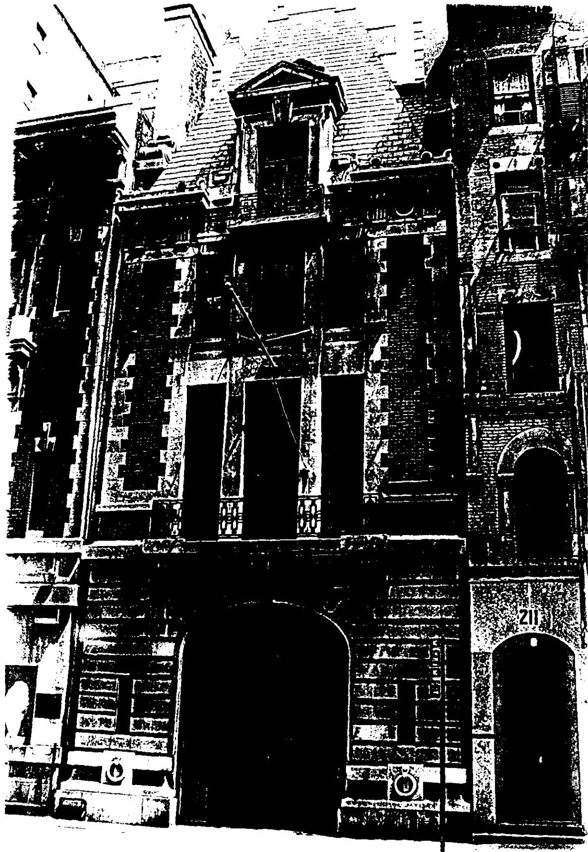
Plate 7. Full elevation, 213 West 58th Street.
