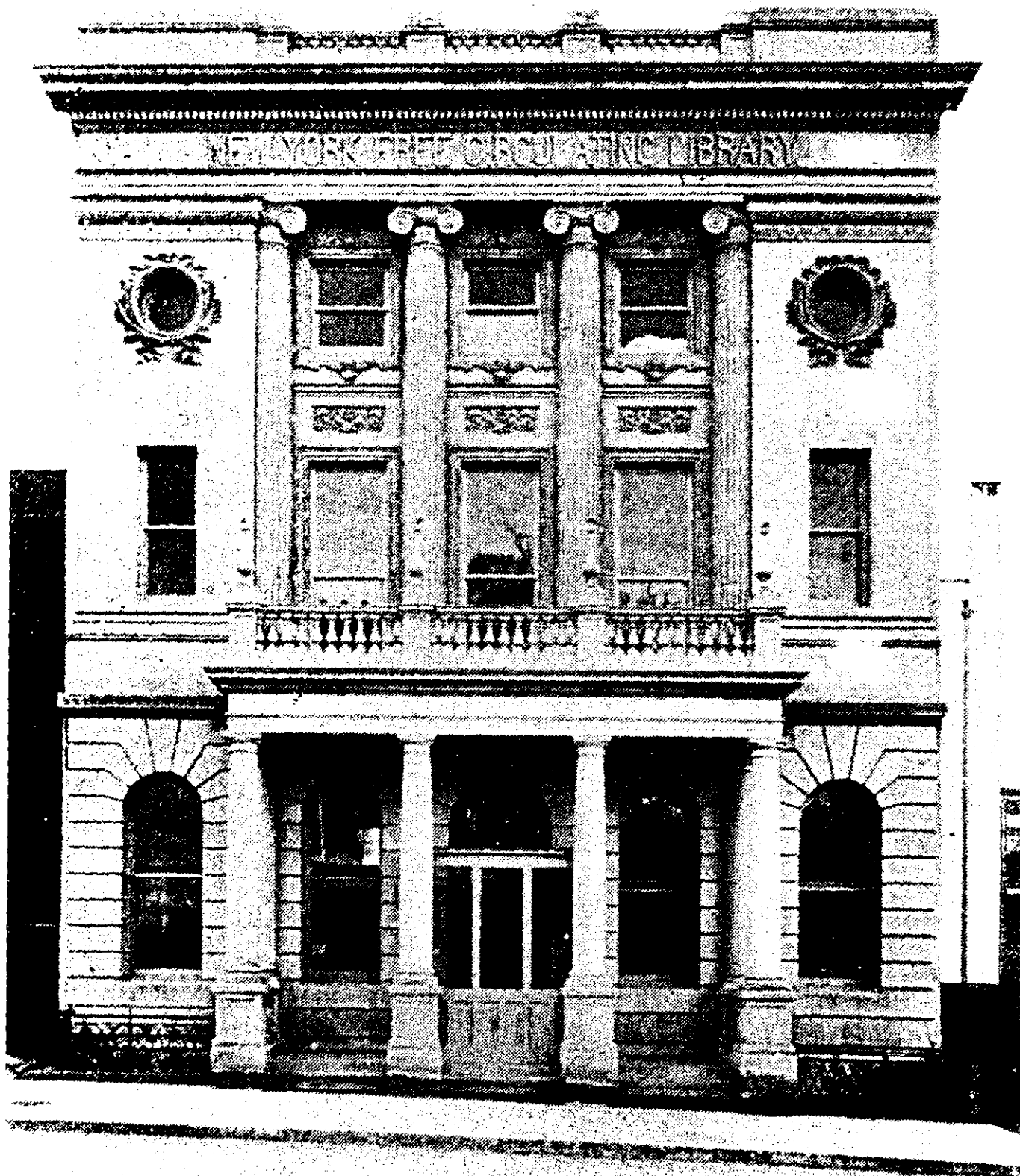
New York Free Circulating Library, Bloomingdale Branch 206 West 100th Street 1898; architect James Brown Lord Photograph from Zeisloft, E. The New Metropolis , 1899.
