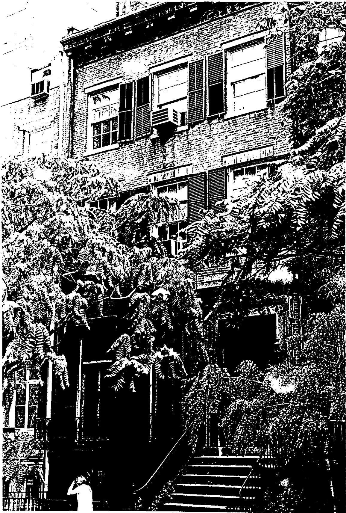
21 West 16th Street Building, 21 West 16th Street (c. 1846)
