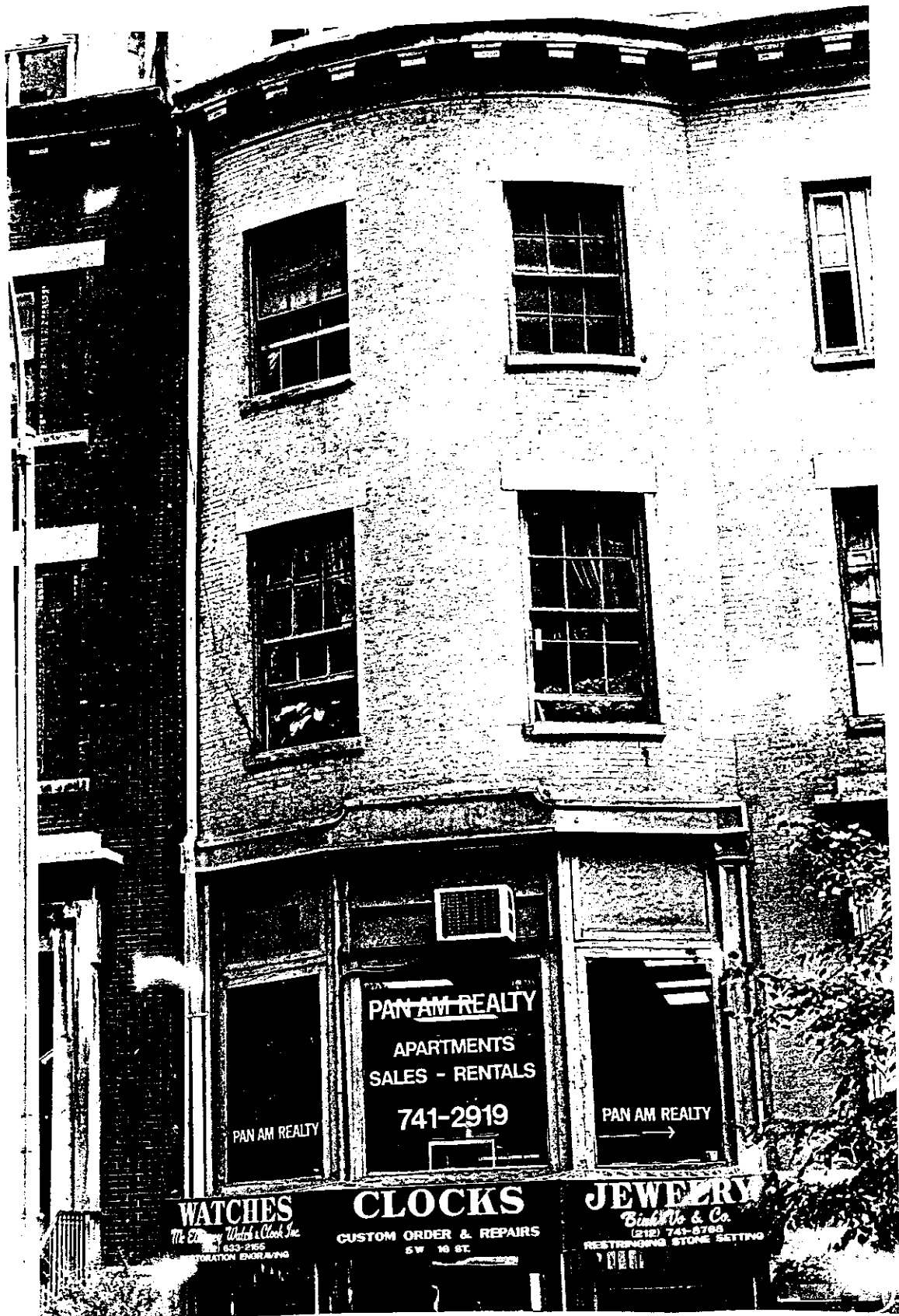
5 West 16th Street Building (storefront detail)
