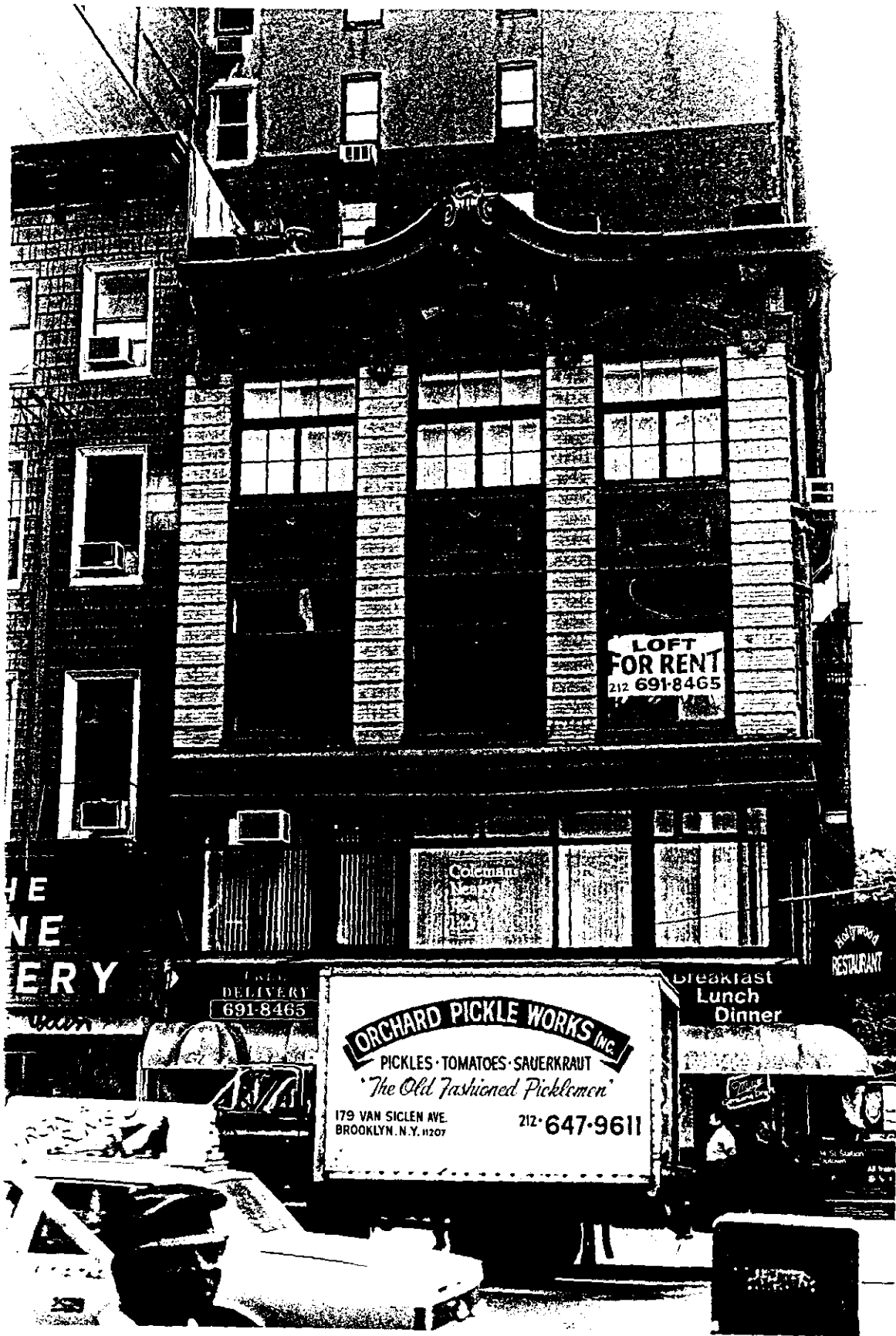
The 574 Sixth Avenue Building, Manhattan. Sixth Avenue facade. 1903-04; architect, Simeon B. Eisendrath. Photo credit: Kevin McHugh
