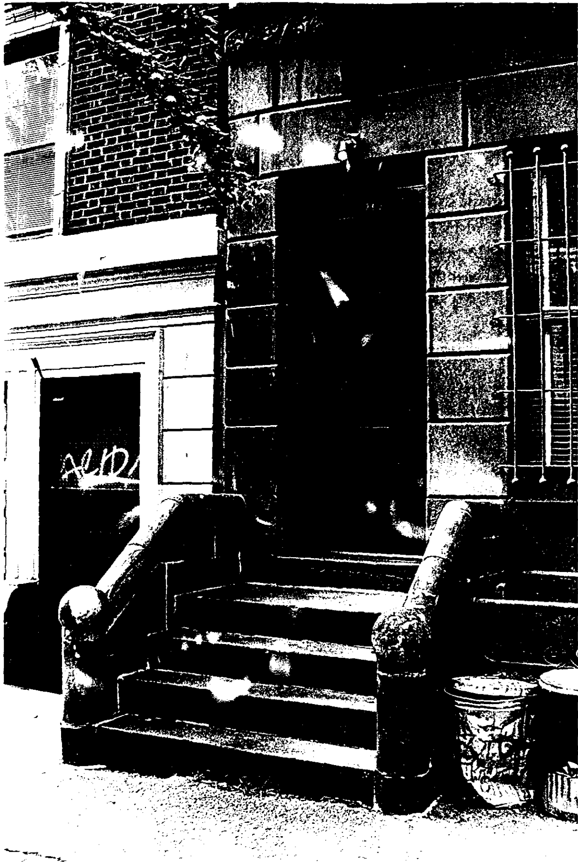
Plate 3. 316 West 85th Street. Detail, entrance.
