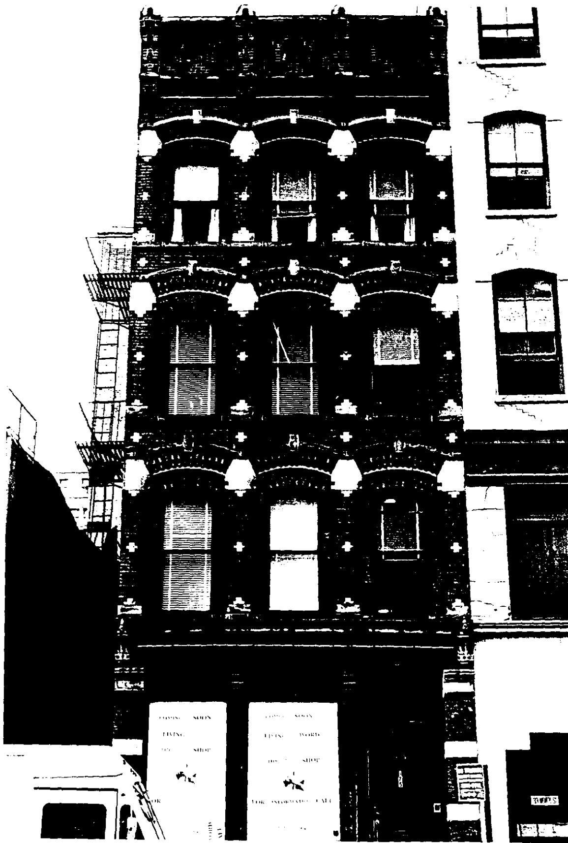
Fig. 2: 175 West Broadway Building
