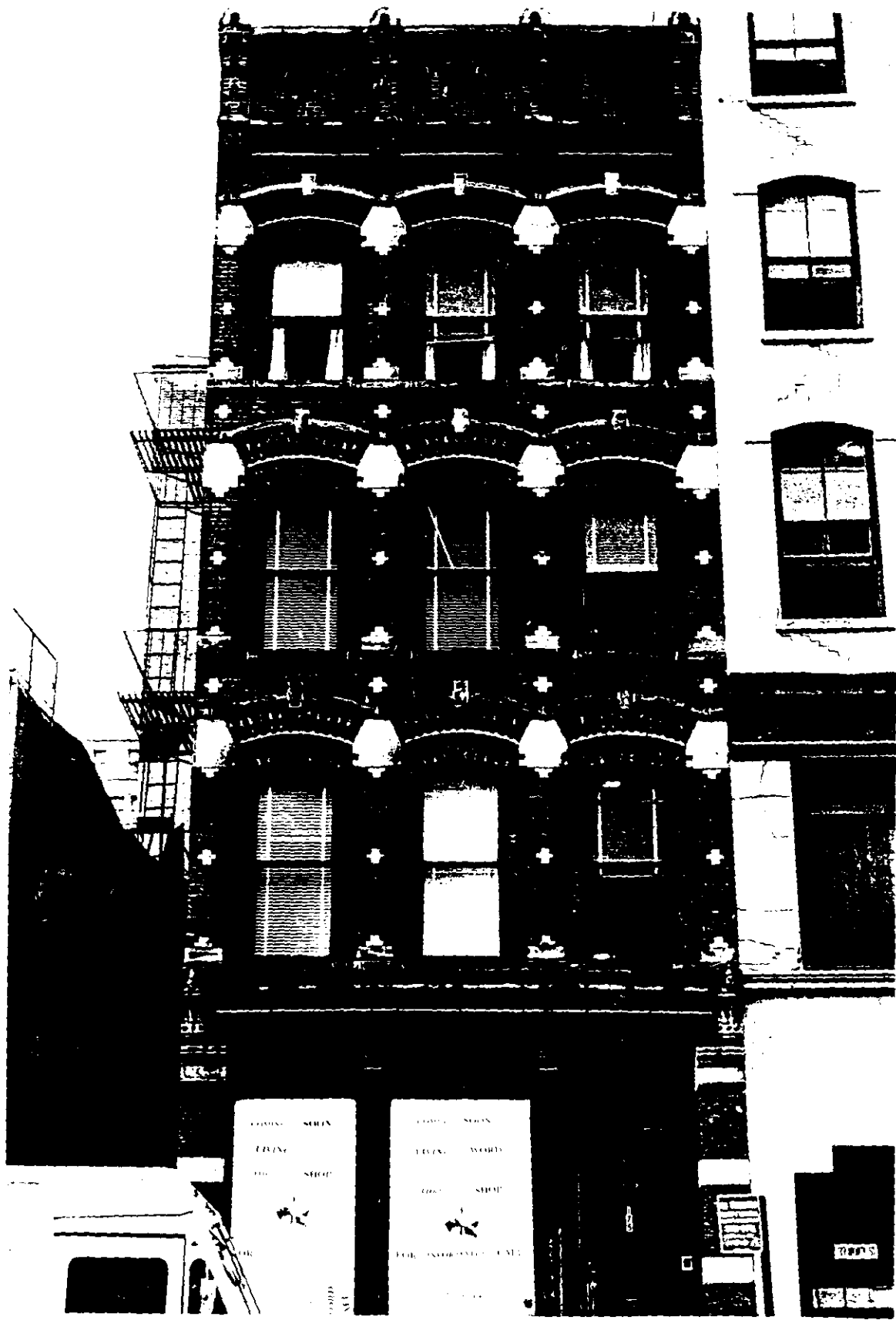
Fig. 2: 175 West Broadway Building
