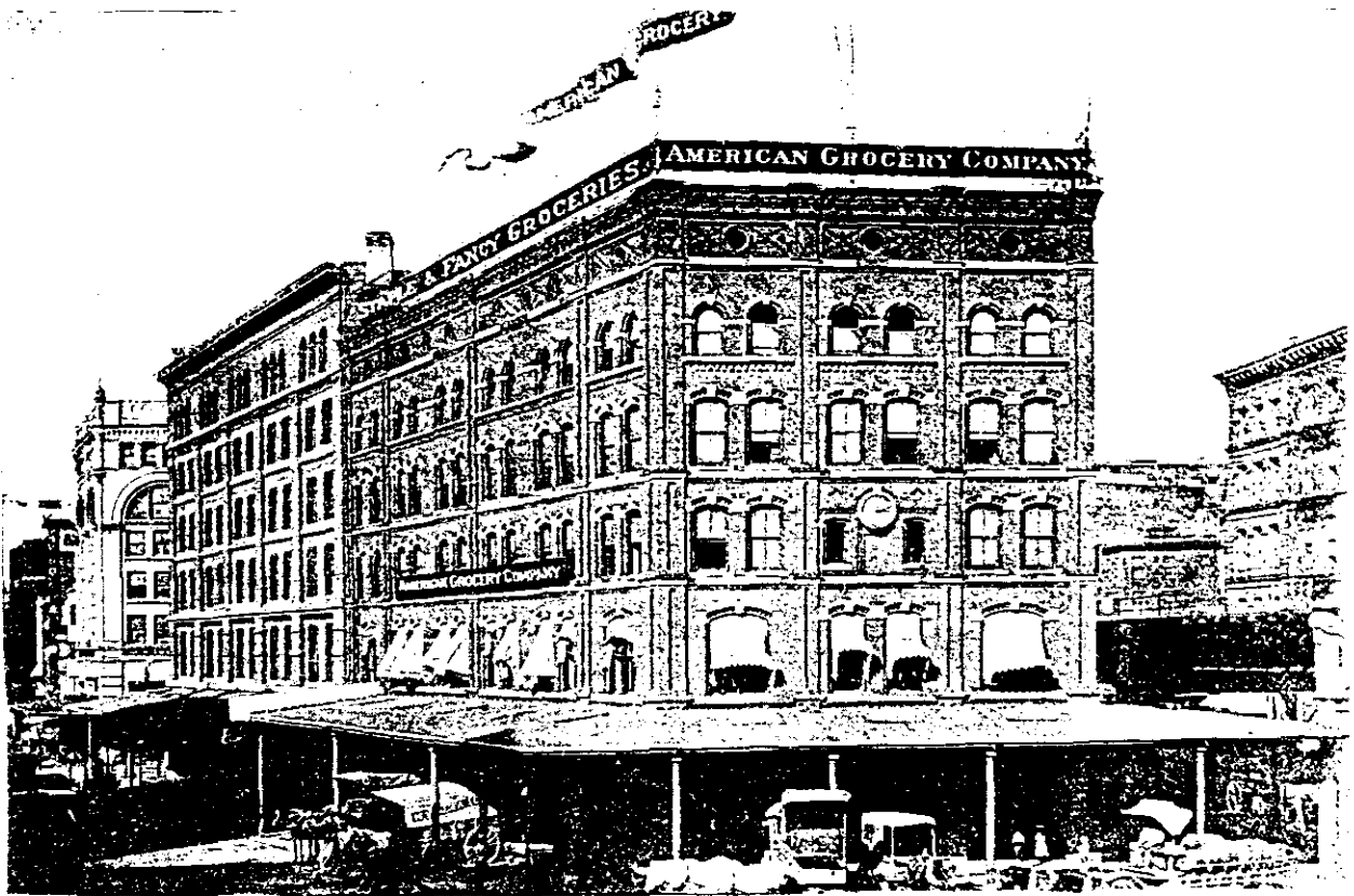
Fig. 6: Warehouse at 16 Hudson Street, C.F. Mengelson, 1873-74 Source: King's Photographic Views of New York
