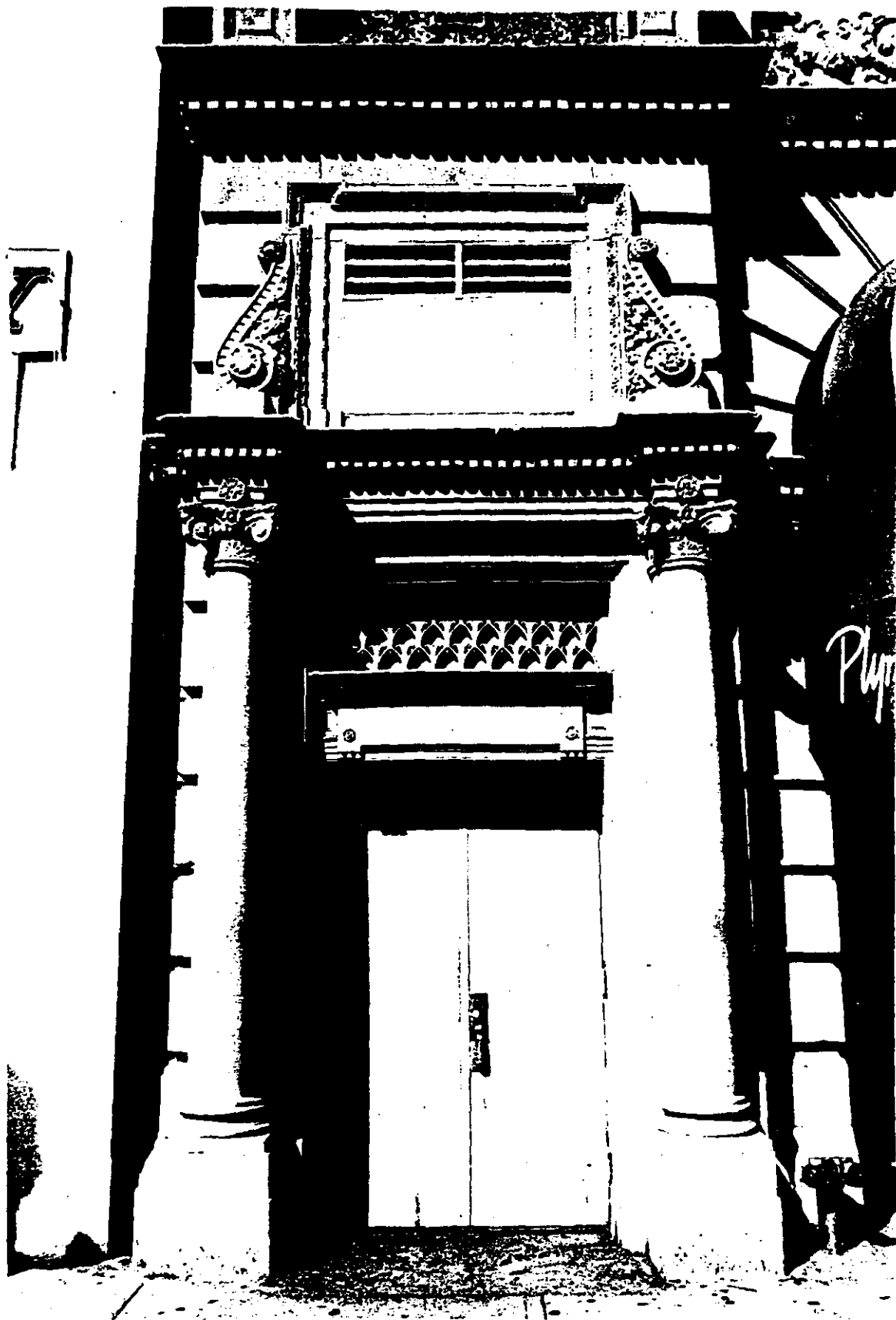
Plate 8. Detail, doorway. Home Life Insurance Company Building. (Carl Forster)
