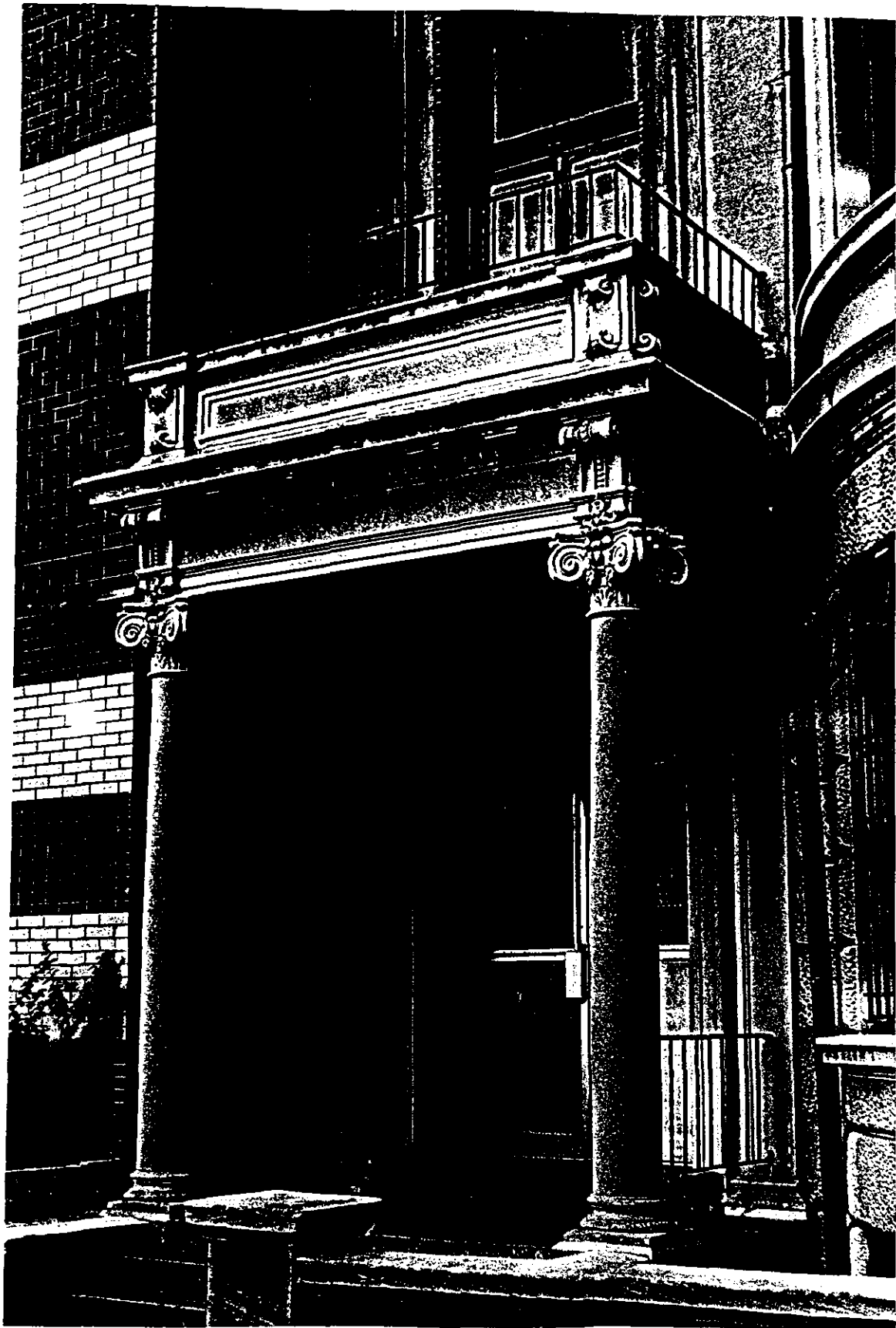
The Prentiss Residence, Detail of Entrance. Photo Credit: Carl Forster.
