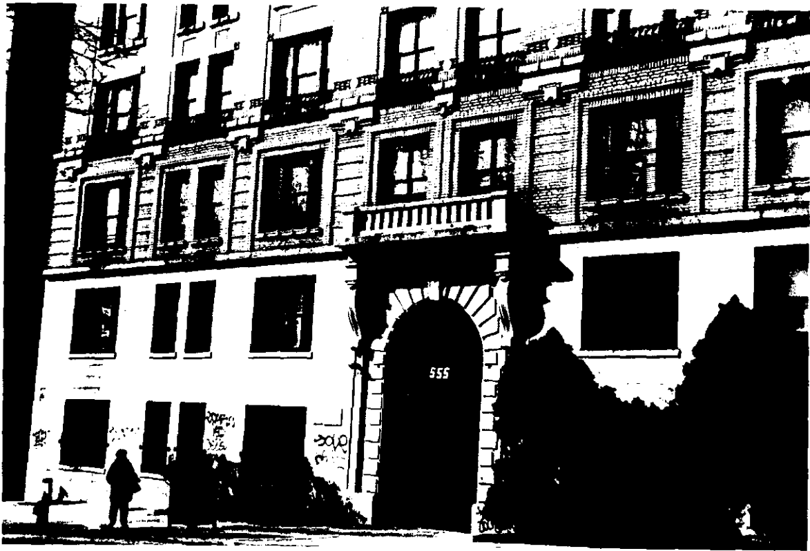
555 Edgecombe Avenue Apartments (Roger Morris Apartments) Detail of entrance
