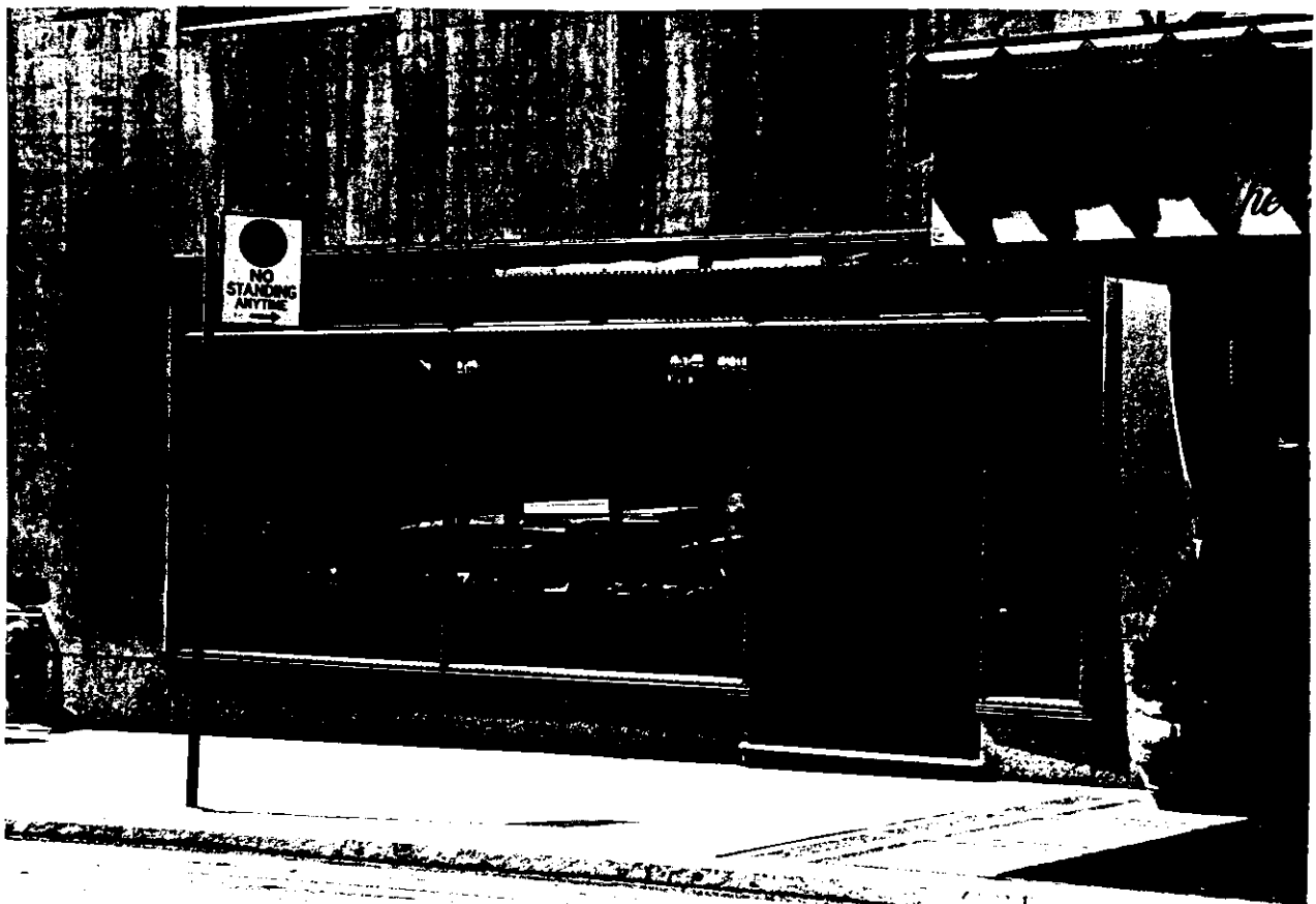
20. Waldorf-Astoria Hotel, storefront, East 50th Street, just east of the Towers entrance
