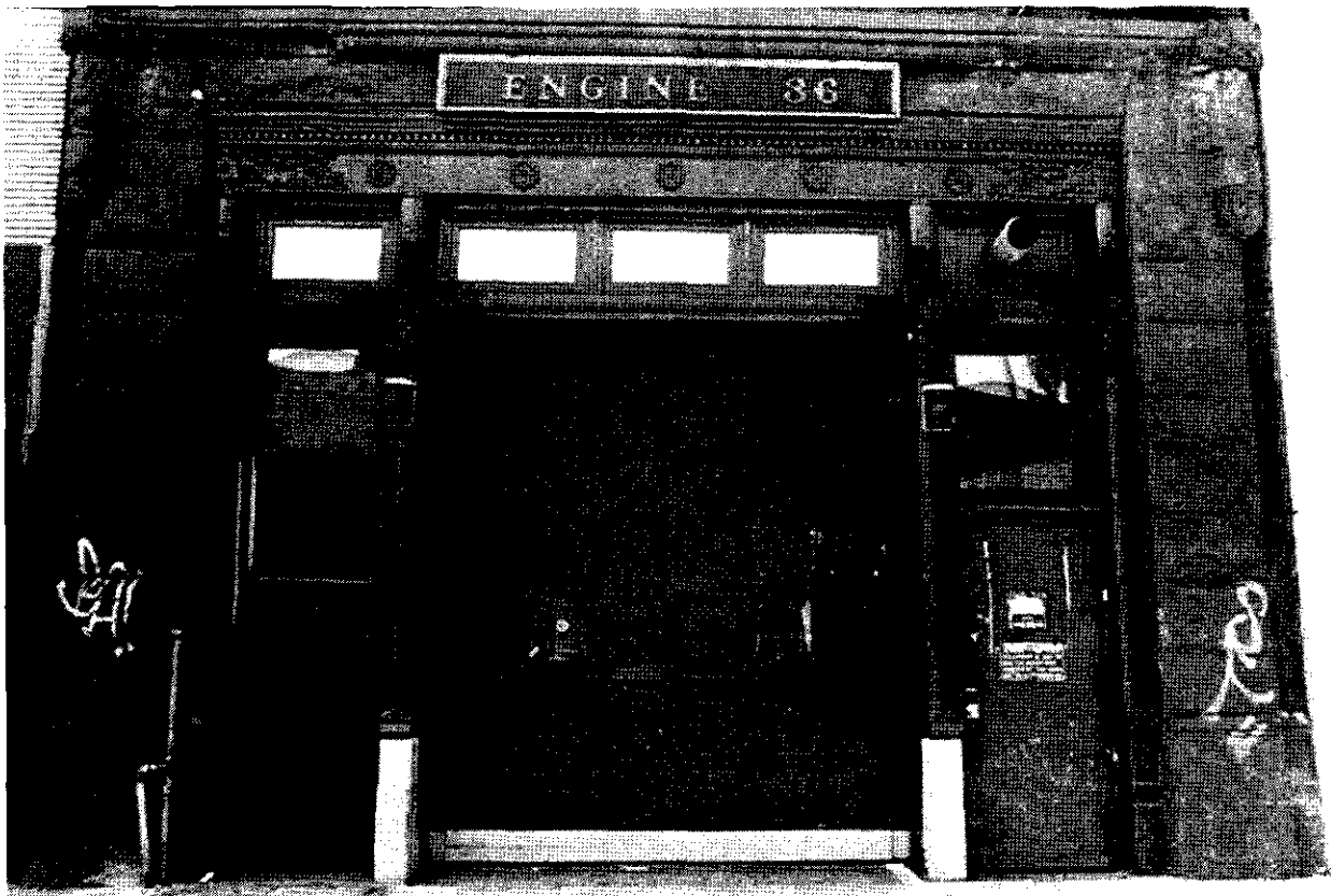
Fire Hook & Ladder Company No. 14 (now Fire Engine Company No. 36) View of base Photo: Carl Forster
