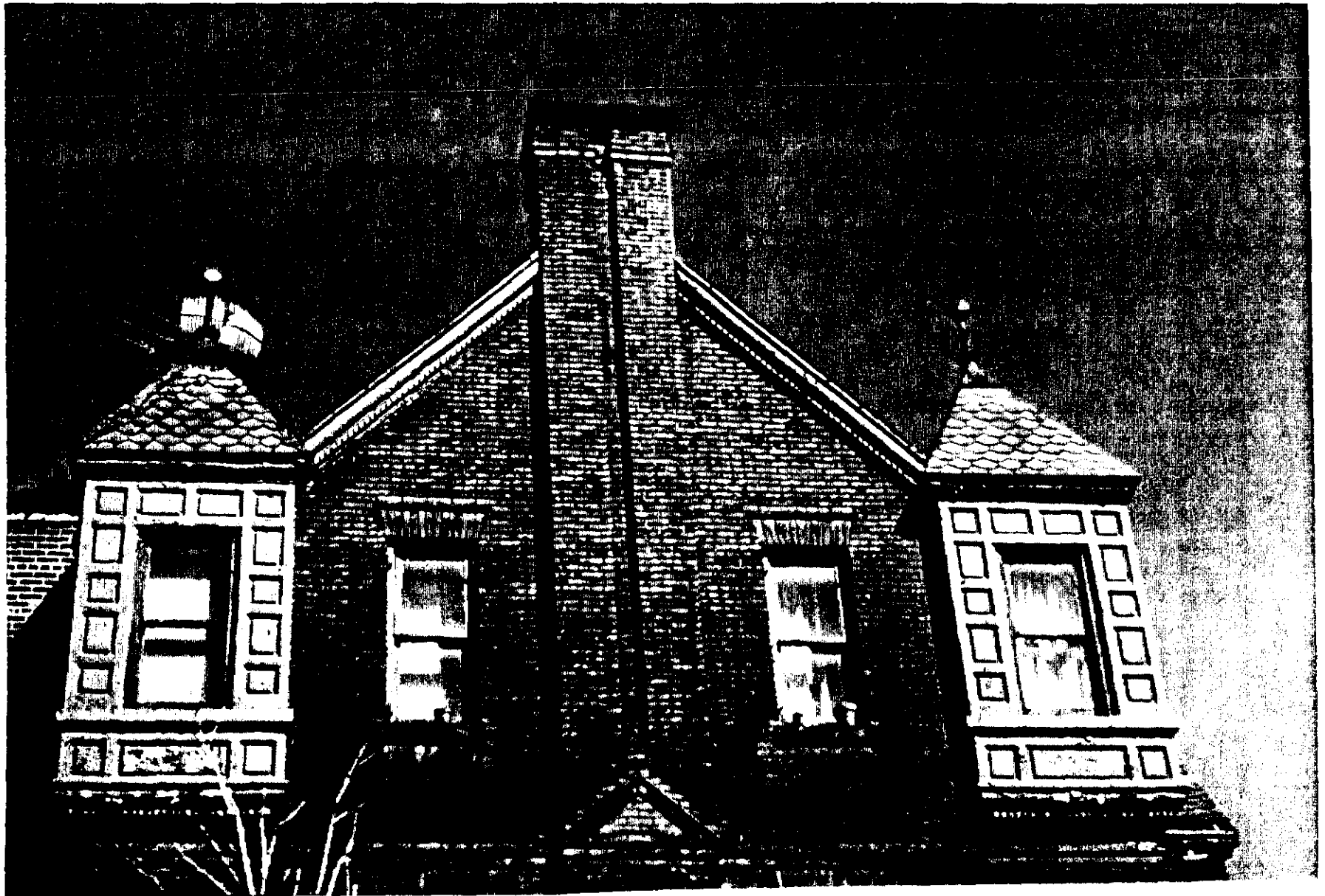
John and Elizabeth Truslow House, 96 Brooklyn Avenue, Brooklyn. Detail of Dean Street gable end and oriels
