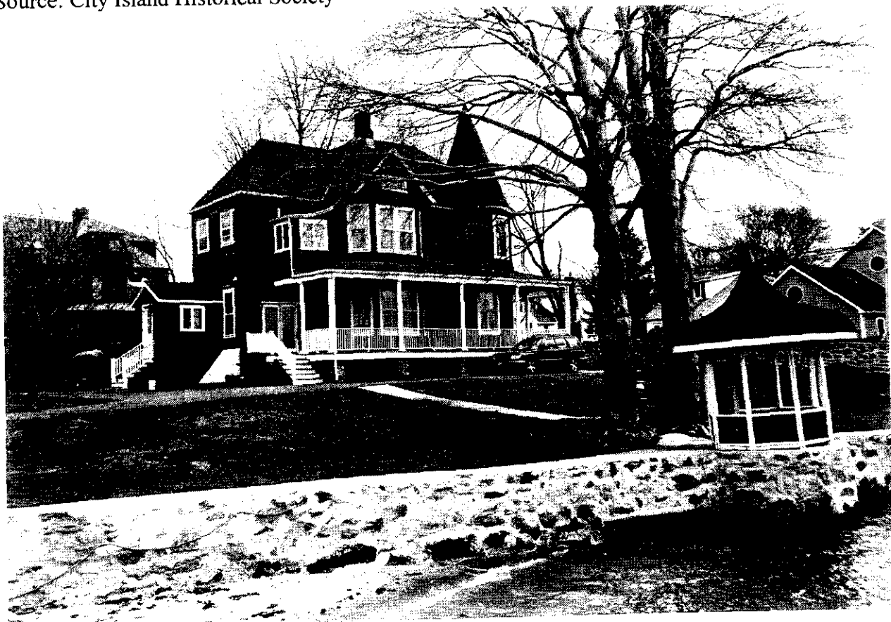
North and West Elevations Photo: Carl Forster
