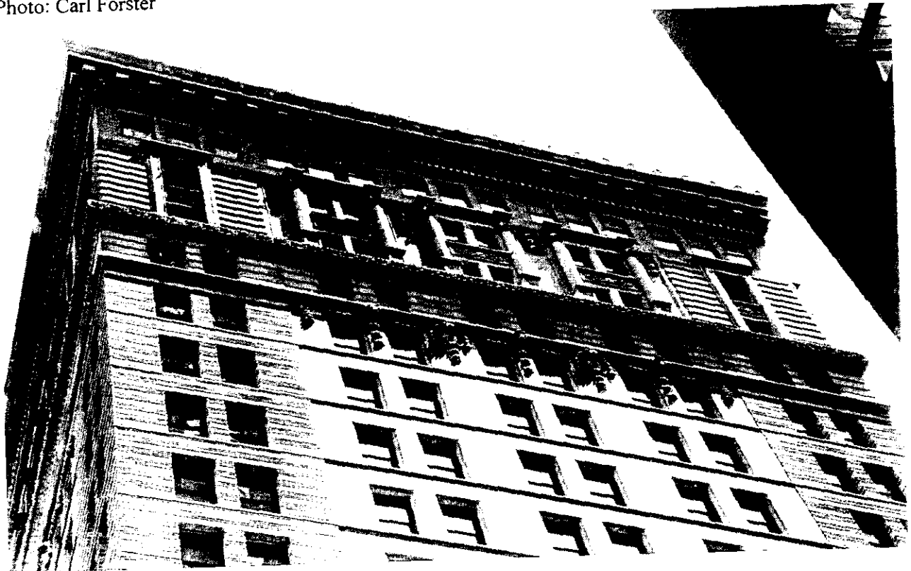
Detail of Cornice, Broad Street Photo: Carl Forster
