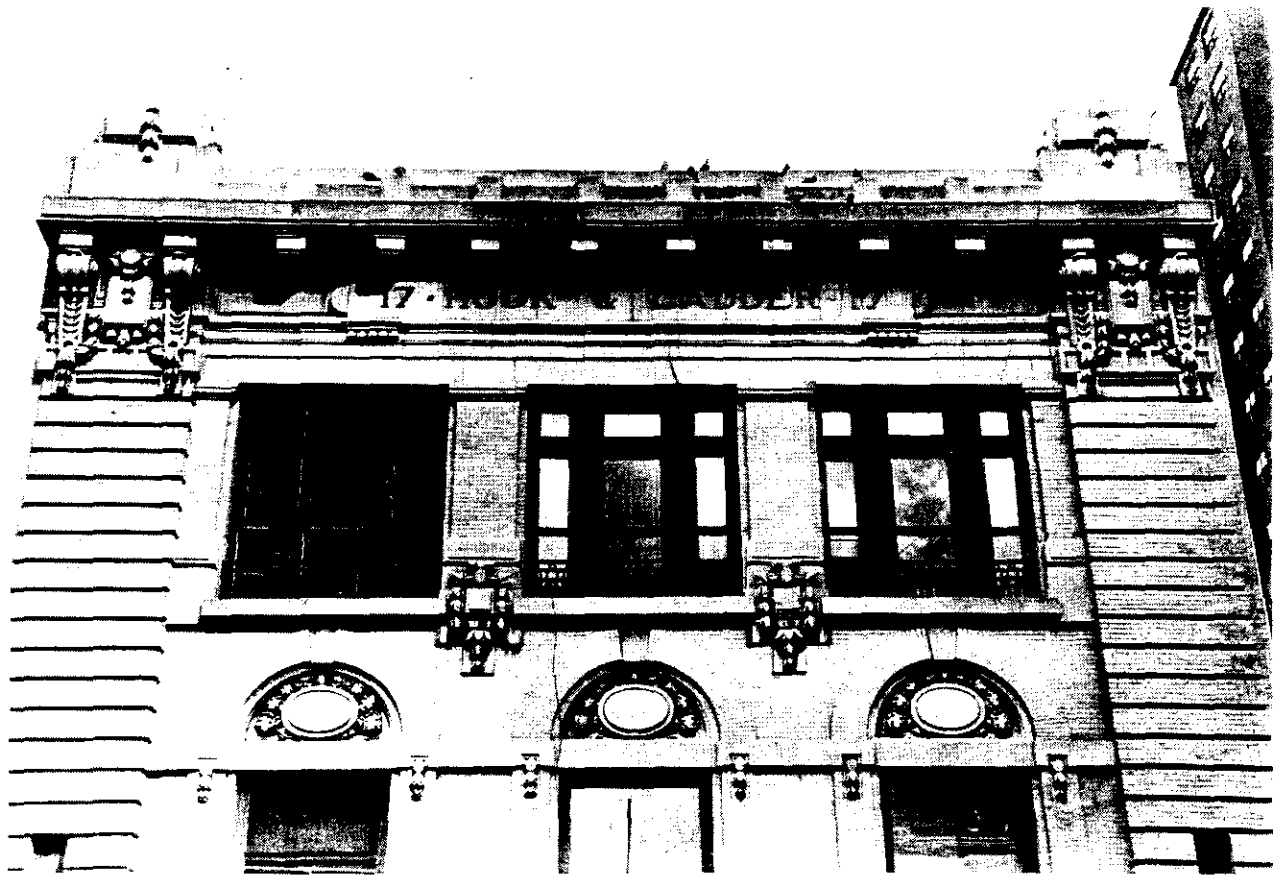
Fire House, Hook and Ladder 17 (now also Engine Company 60) Details
