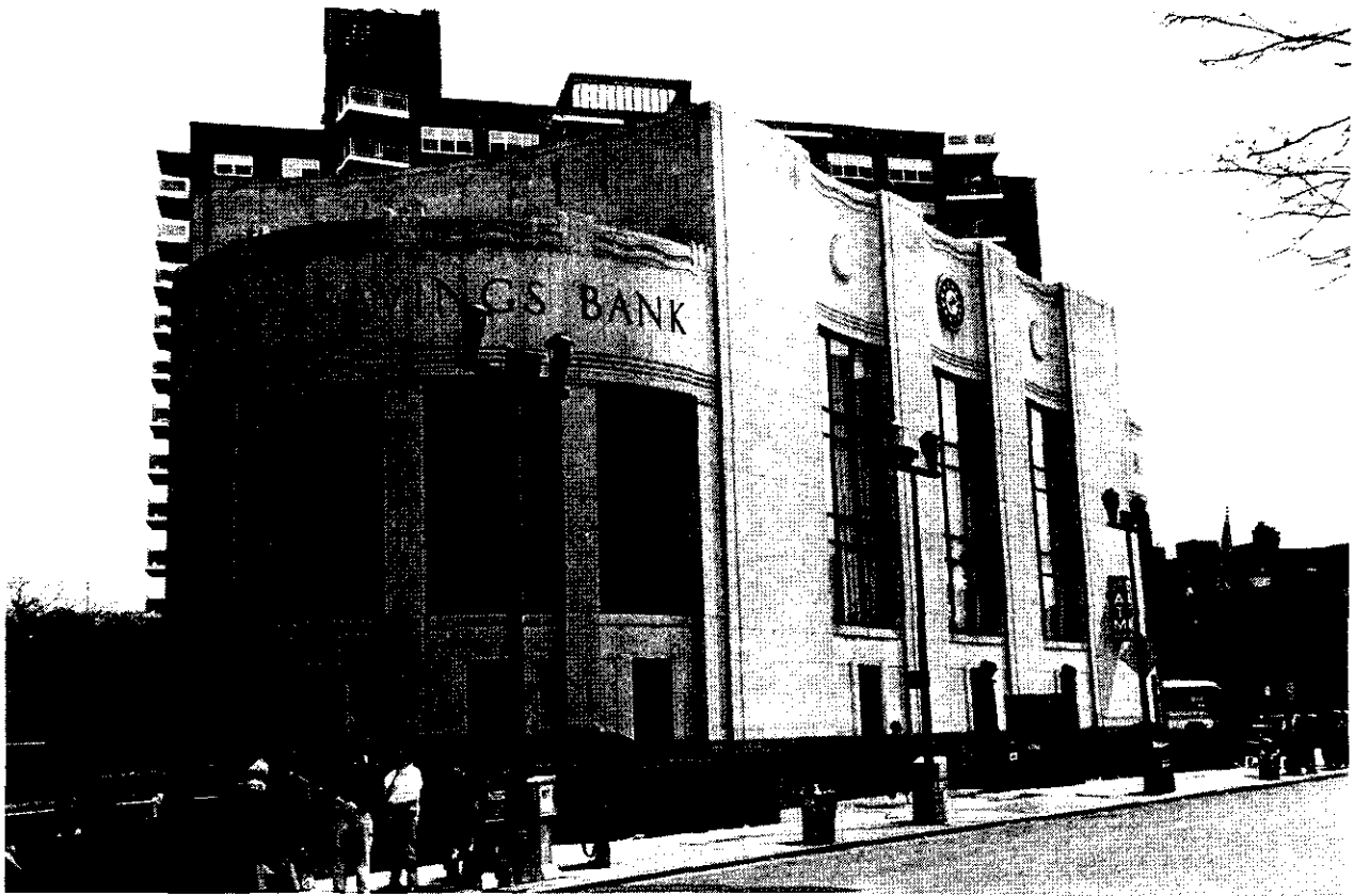
View from the west
