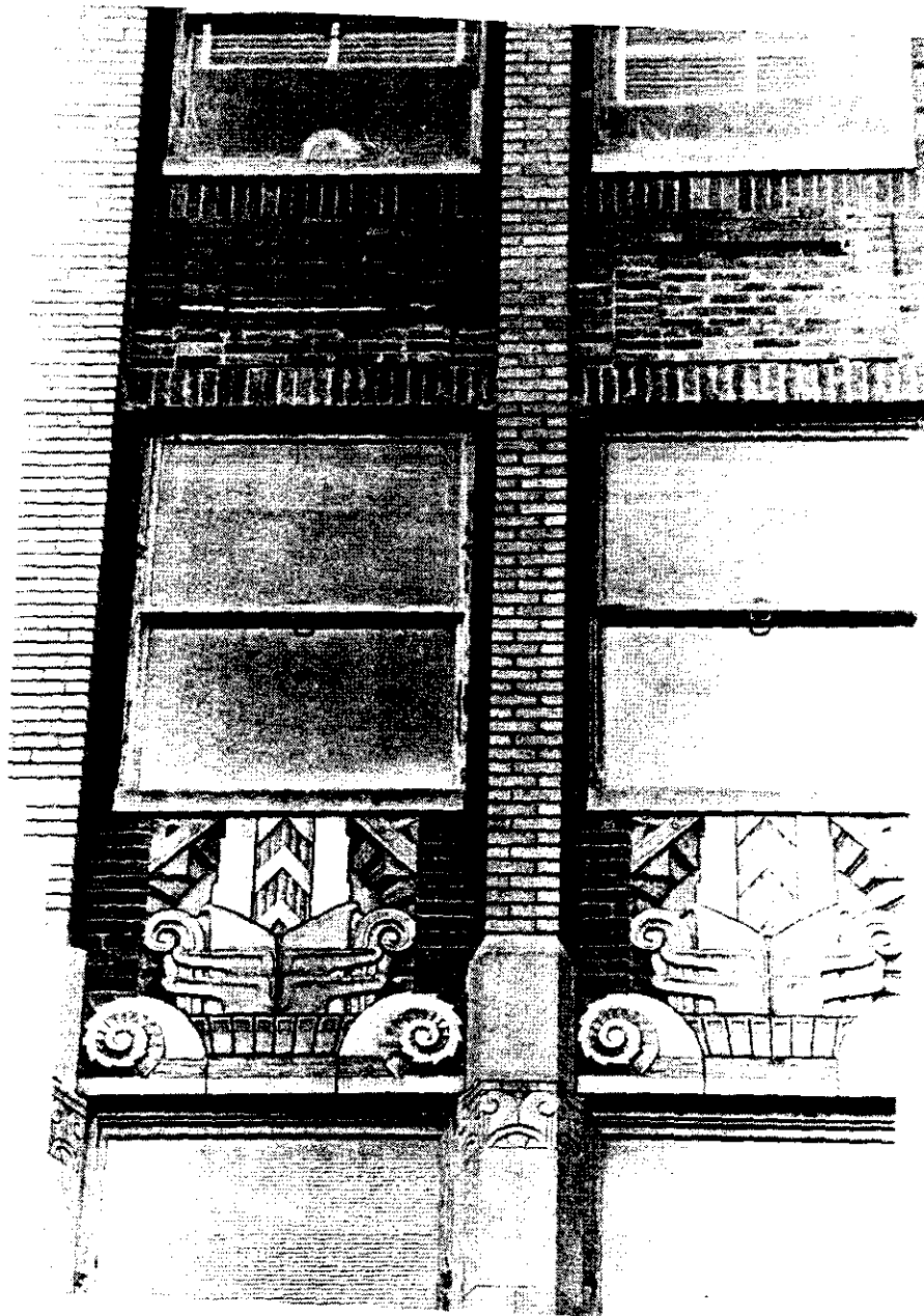
(Former) Suffolk Title Guarantee Company Building Detail, terra-cotta panels Photo: Bill Neeley
