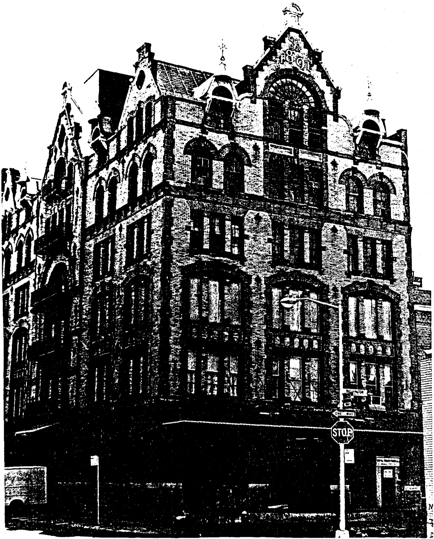
FLEMING SMITH WAREHOUSE 451-453 WASHINGTON STREET
